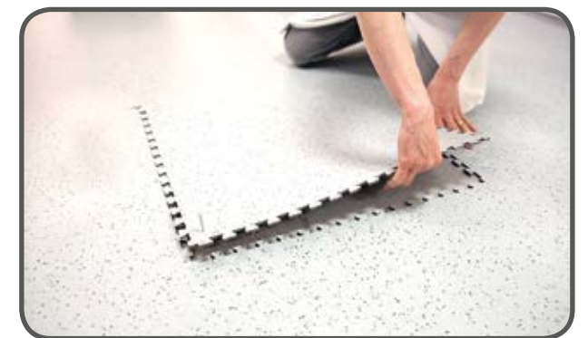
Damaged tile out / New tile in
